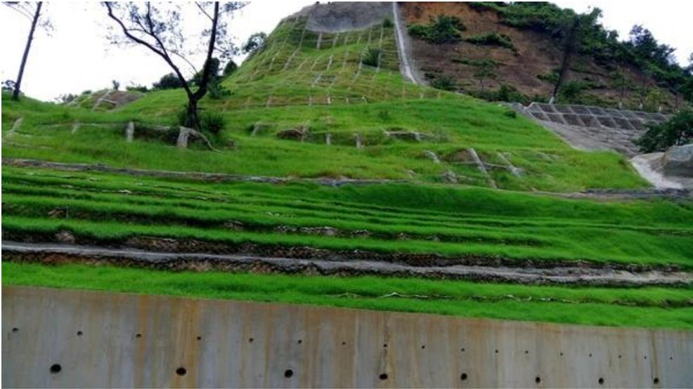
Figure 7 Reinforcement and maintenance is conducted on potentially dangerous slopes.
